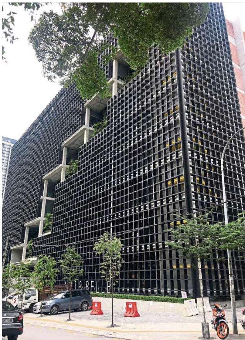
Unique feature: Diagonally-stacked and landscaped open atriums through the building's centre promote cross ventilation – not to mention an interesting aesthetic touch. — Photos: SAM THAM/The Star
